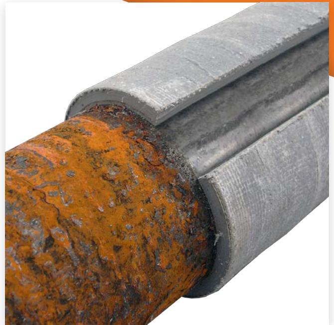
Section removed showing uncorroded pipe
