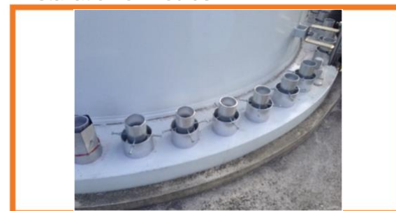
Installation of moulds
