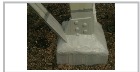
Concrete “Muff” after TM198 application
