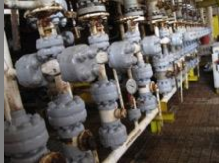
After minimal surface preparation and application of TM198
