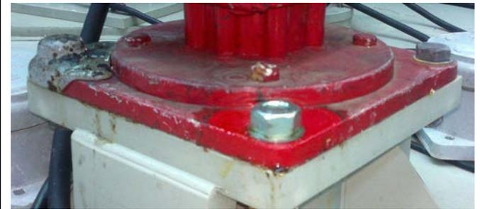
Oxifree coating peeled off from the nut on the right front of the agitator. Compare to the corroded nut at the back, right. Nuts made of stainless steel.
